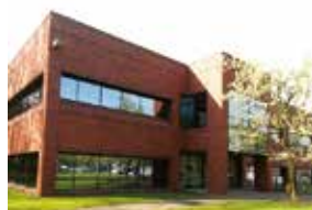
FLIR Systems, Portland
